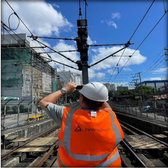
Overhead Catenary System
