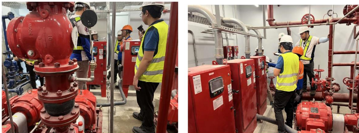
19 July 2024 : Testing and Commissioning of Fire Pumps (Redemptorist Station)
