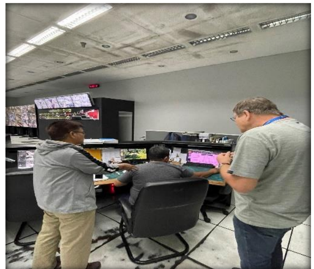
OCC Workstation for SCADA
