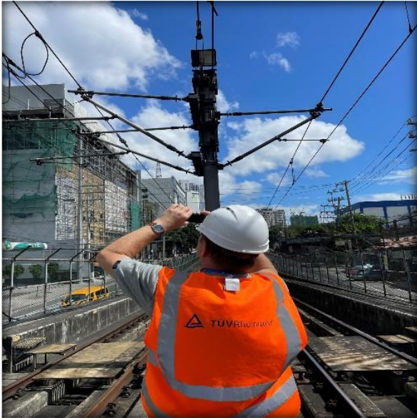
Overhead Catenary System
